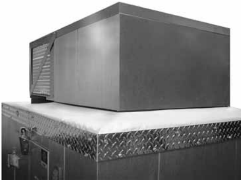
Exterior view of roof-curb mounting technology for drop-in refrigeration outdoor installations.
